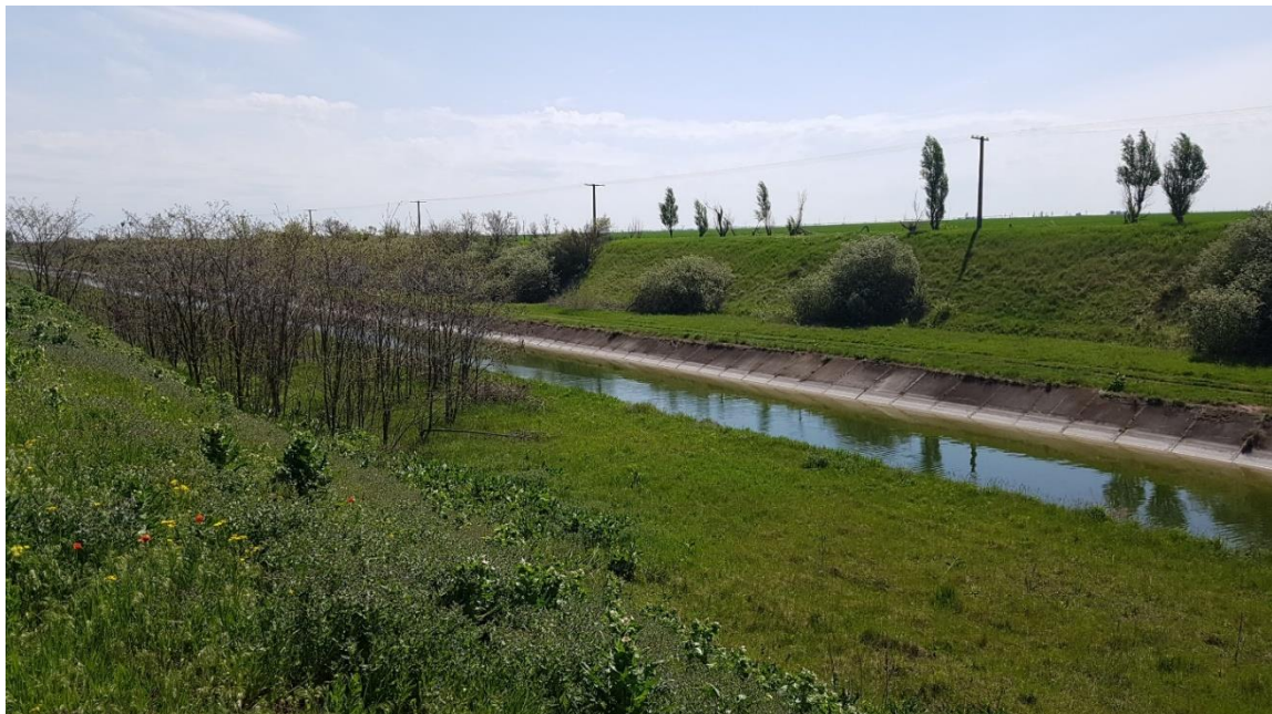
Figure 7-1: Drainage / Irrigation Channel
